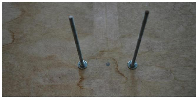
Figure 12. Grip the threaded rods using nuts and washers
