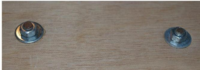
Figure 13. Turn the wooden base upside down and grip the threaded rods using nuts and washers
